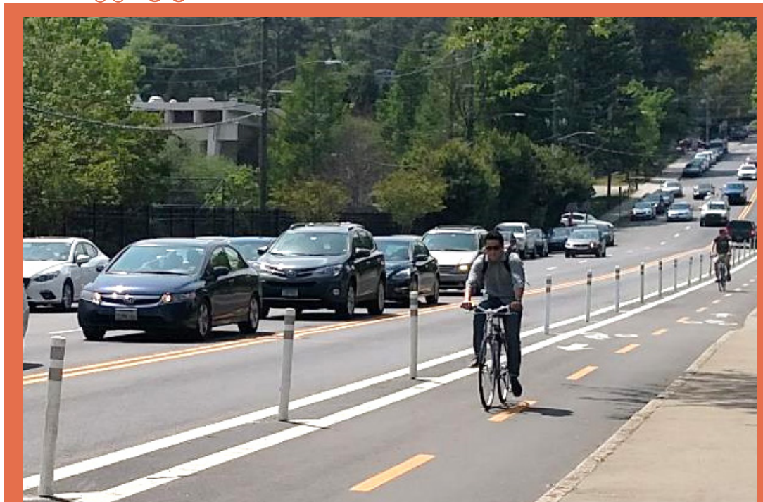
Example of Two-Way Separated Bicycle Lane, 10th Street NW, Atlanta, GA
