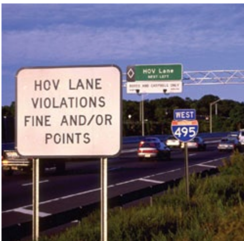
Future I-495 Express Lane, Virginia
