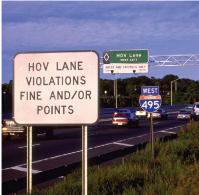
Future I-495 Express Lane, Virginia
