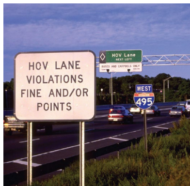
Future I-495 Express Lane, Virginia
