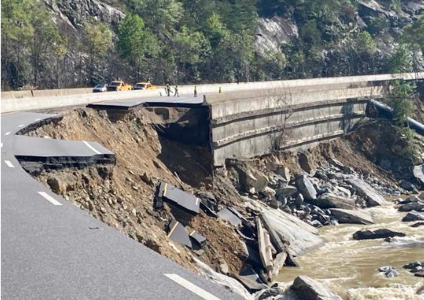
Figure 4.8: Damage to I-40 in Haywood County resulting from Hurricane Helene (credit: NCDOT)
